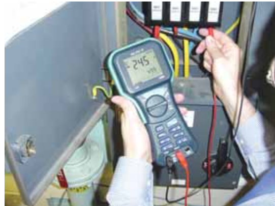
Checking the circuit continuity by multimeter
